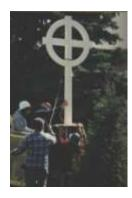
What we see as that little cross at the top of the steeple surprisingly stands 6' high. And, like a tree with its roots, there is an additional 6' anchoring it to the *inside* of the steeple.
