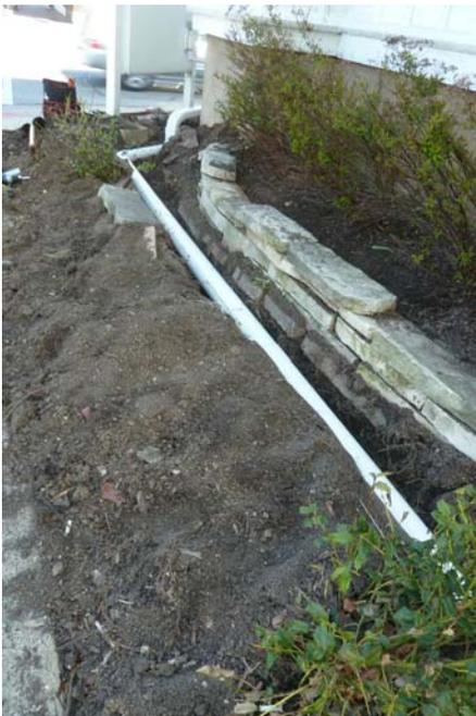
So we did the next-best thing and buried a perforated pipe along the top of the sloped area, distributing the water across the 50' width.
