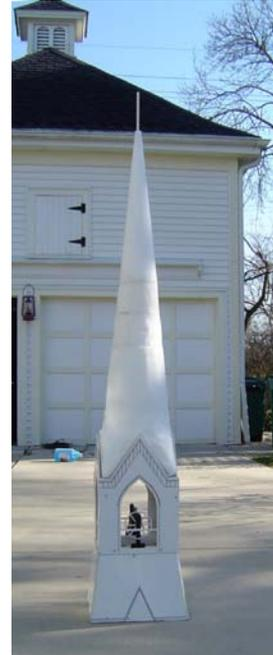
The shape of the bottom of the steeple is rather complex - the pointed tops of the sides of the belfry form dormers into the cone-shaped steeple, and each corner kind of sweeps out from the 12" diameter circular shape to a 12" square bottom.
